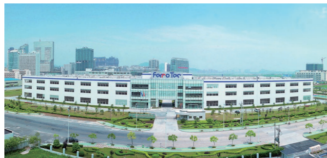
Hangzhou Dahe Thermo-Magnetics Co., Ltd. Plant 2 (Hangzhou)
