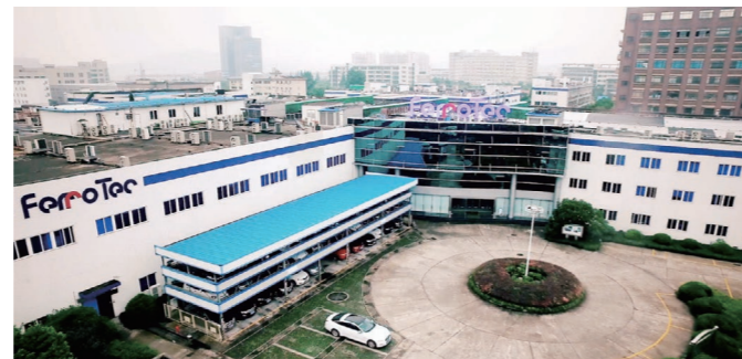
Hangzhou Dahe Thermo-Magnetics Co., Ltd. Plant 1 (Hangzhou)
