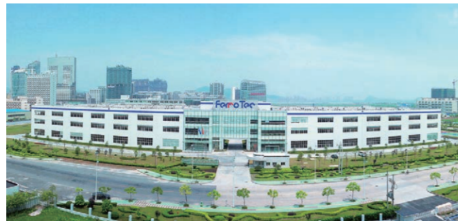
Hangzhou Dahe Thermo-Magnetics Co., Ltd. Plant 2 (Hangzhou)
