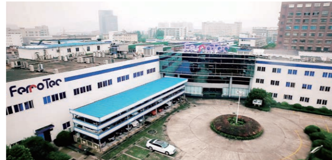
Hangzhou Dahe Thermo-Magnetics Co., Ltd. Plant 1 (Hangzhou)
