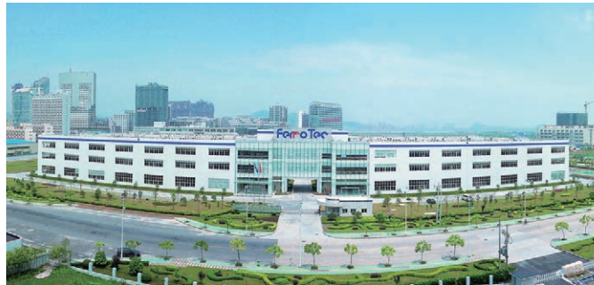
Hangzhou Dahe Thermo-Magnetics Co., Ltd. Plant 2 (Hangzhou)
