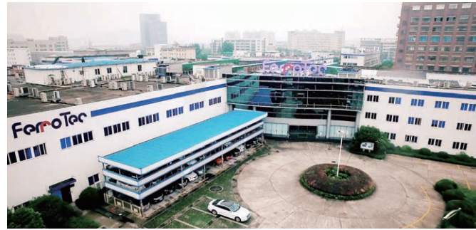
Hangzhou Dahe Thermo-Magnetics Co., Ltd. Plant 1 (Hangzhou)
